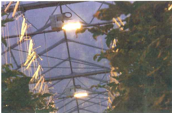
Up to 60% of the light needs to be caught by the reflector and directed back toward the plants.
