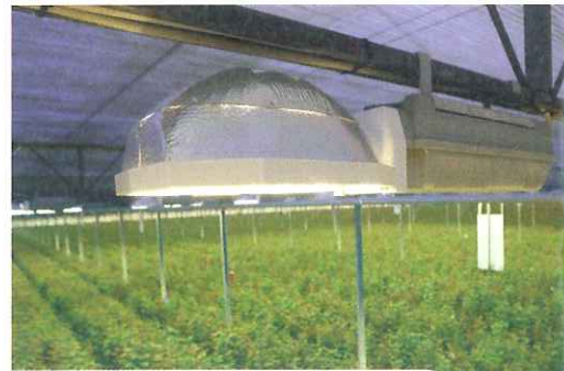
Up to 60% of the light needs to be caught by the reflector and directed back toward the plants.
